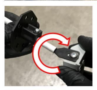
7. Insert the injection assembly through the injection port, until it meets the duct. While using a level, ensure that the 'UP' arrows are pointing vertically up as shown. Note: the vertical orientation of these planes is important to help prevent condensation from draining into the HVAC system
