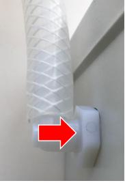
5. Secure the assembly from inside the cabinet with the sealing nut provided. Tighten the nut to ensure that the seal on the nut creates a water tight seal against the interior wall of the cabinet:
