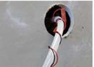
5. Slide the cord management sleeve over the tube and wire.
