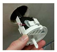
3. Screw in the two screws until you feel the plastic snug towards the drywall.
