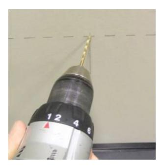
3. Using an appropriate step drill, enlarge the pilot hole to a 7/8" diameter hole.
